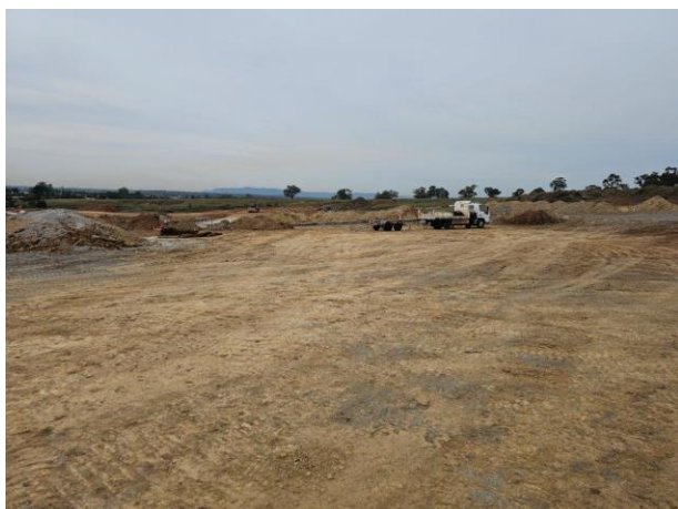
Photograph 15: From boundary of Lots 126 and Lot 127, (near BHQ13), facing south.
