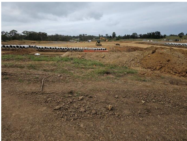
Photograph 13: From boundary of Lots 122 and Lot 123, (near BHQ11), facing north.
