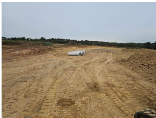
Photograph 16: From boundary of Lots 126 and Lot 127, (near BHQ13), facing west.
